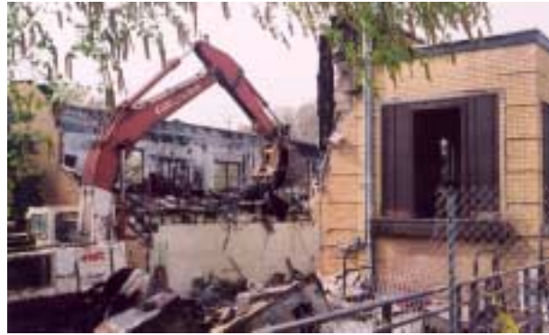
Cafeteria during demolition process
